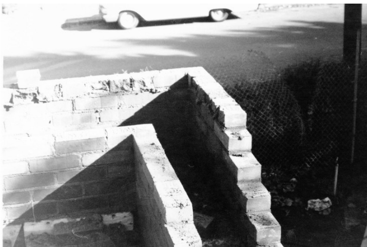
Walls of the BBC deck under construction
