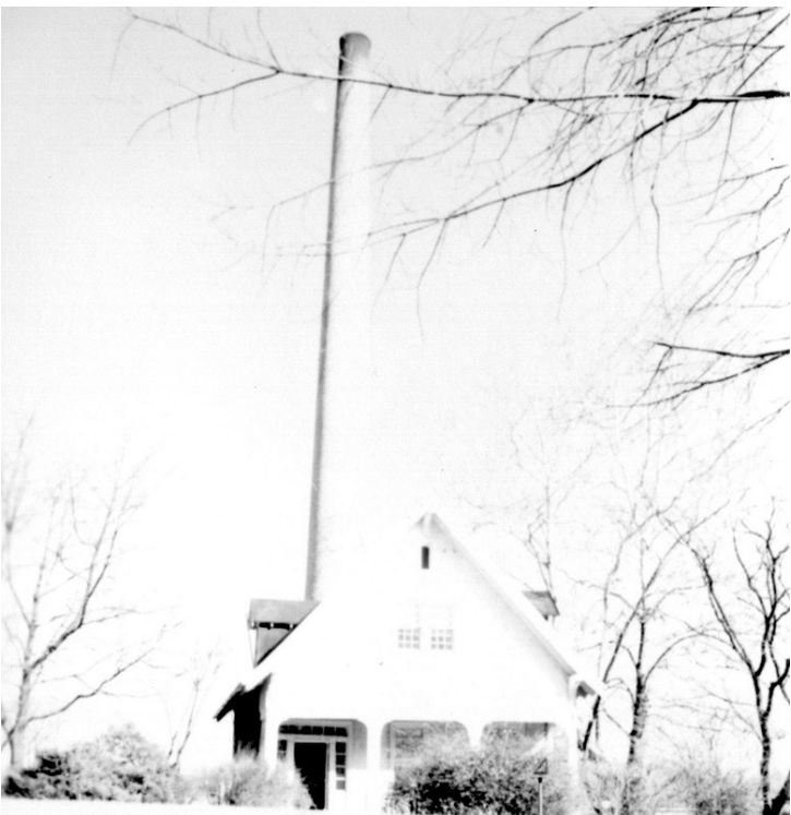
Old heating plant, 1940-1950
