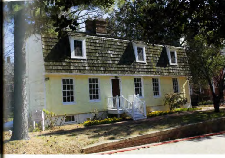
Chancellor Johnson House
