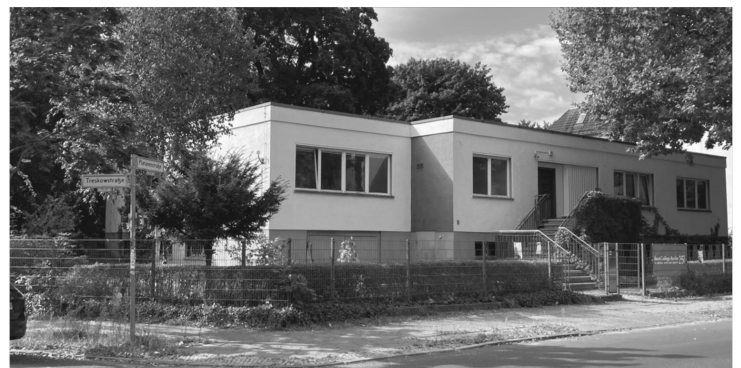
Teaching building (former residence of the cultural attaché of the United States) (photo: Helen Felbek)
