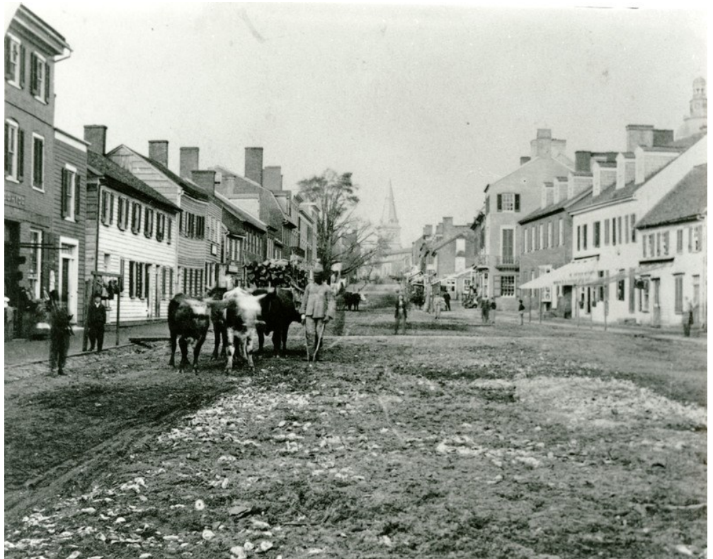
Main Street, Annapolis, ca 1870. The second building from the front on the right currently is the home of Kilwins, while the buildings on the left have been replaced by the building now occupied by CVS. Preserve is located further down the street.
