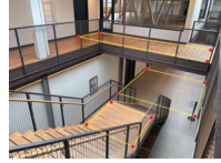
AREA TRACKING Fully Programmable Regional Intrusion Detection
