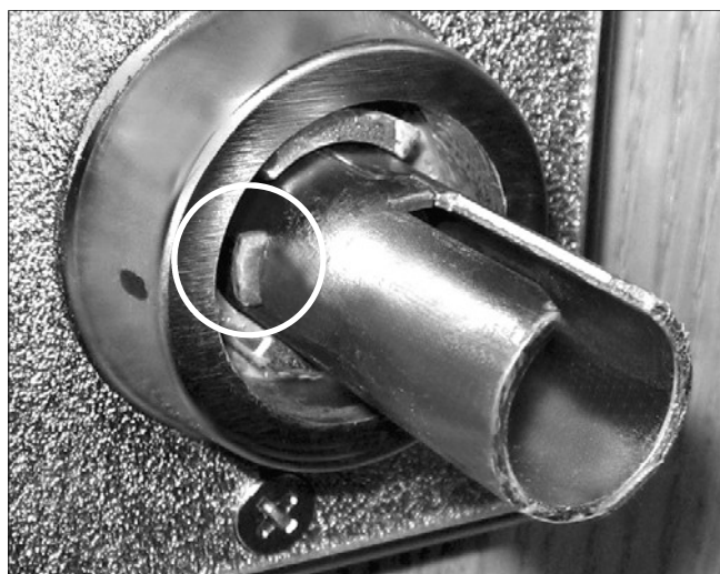
FIG. 6: PUSH IN LEVER CATCH (CIRCLED)
