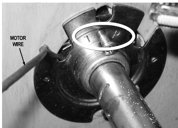
FIG. 12: INSIDE ROSE PLATE INSTALLATION
