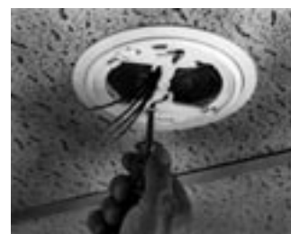
Figure 2. Install detector.
