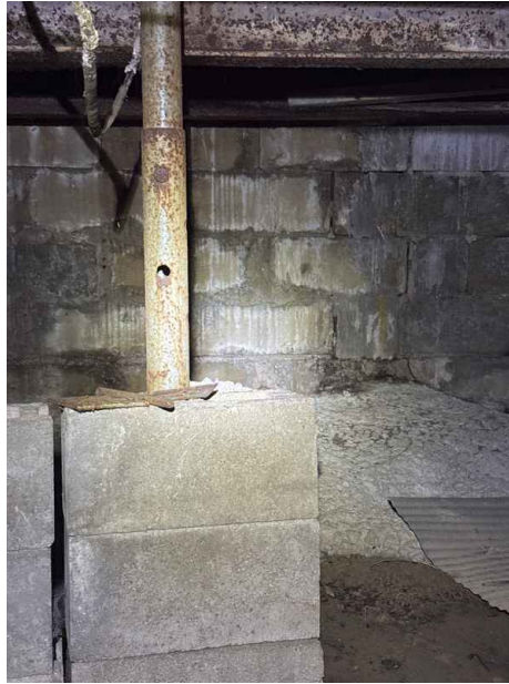
Basements & Crawlspace: Crawlspace
