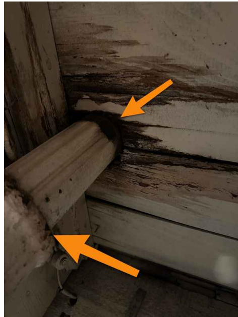
Basement Laundry Room
