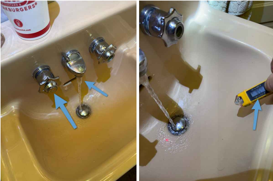
2nd Floor Bathroom
