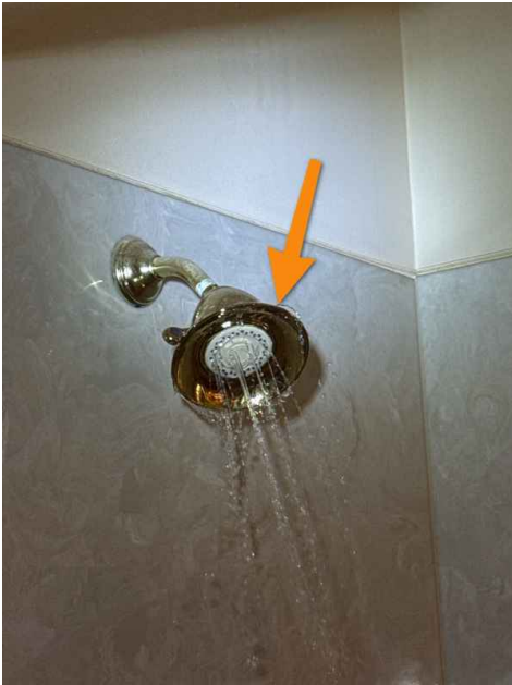
1st Floor South Bathroom
