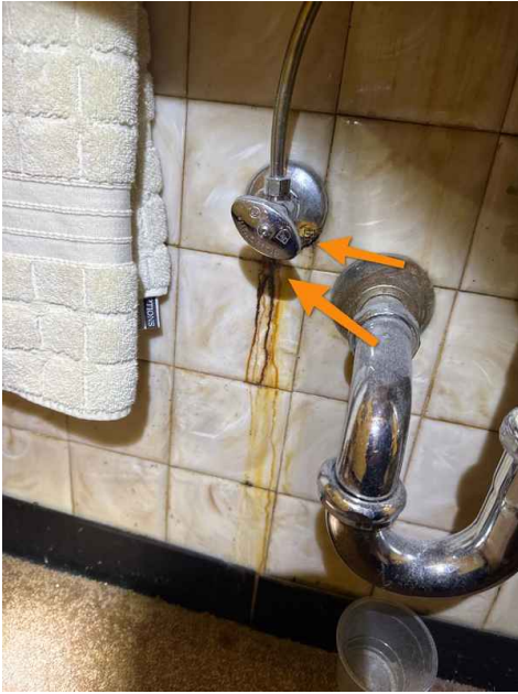
2nd Floor Bathroom
