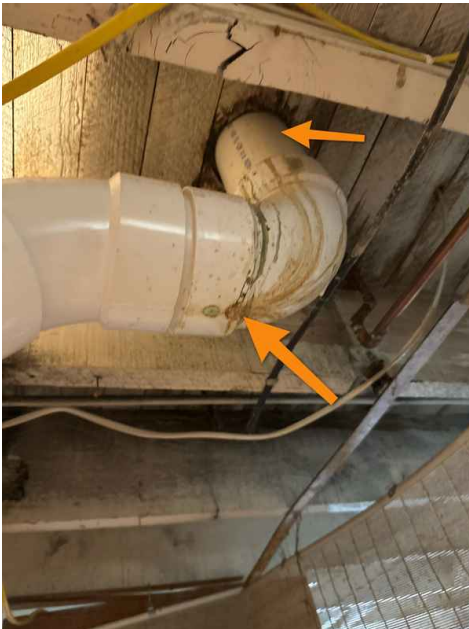
Basement Laundry Room
