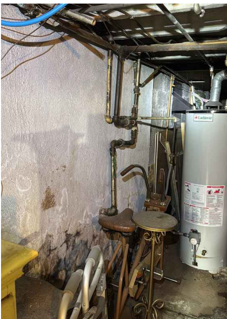
General: Inspection Method Visual
