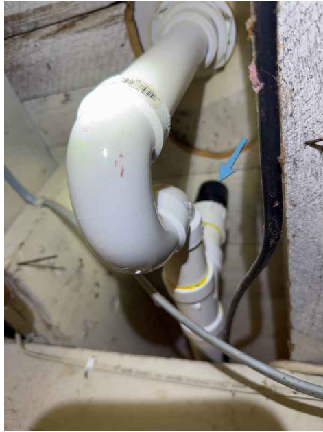
Basement Laundry Room
