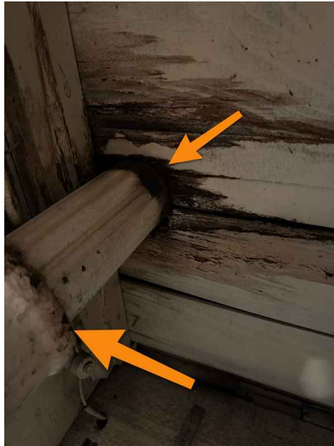
Basement Laundry Room
