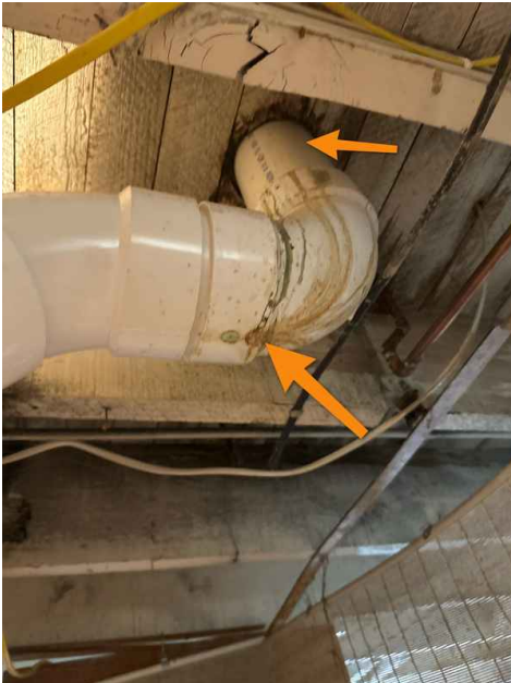
Basement Laundry Room
