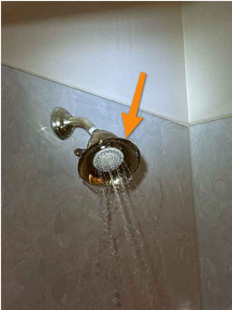
1st Floor South Bathroom
