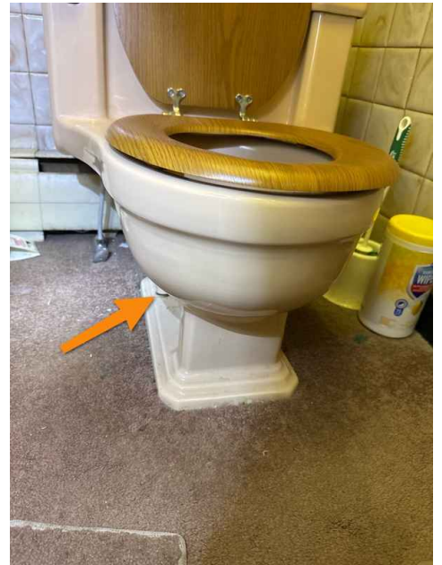
2nd Floor Bathroom
