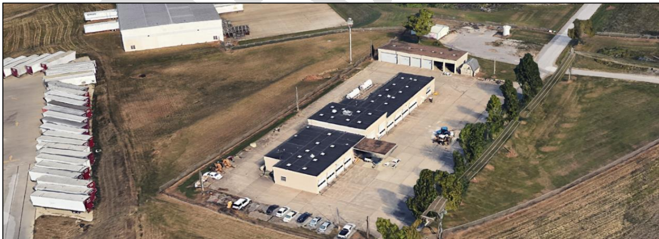
Figure 2-24 – Airport Maintenance and Equipment Storage Facilities
