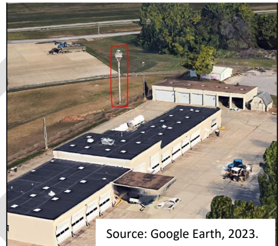
Figure 2-8 – EVV Rotating Beacon
