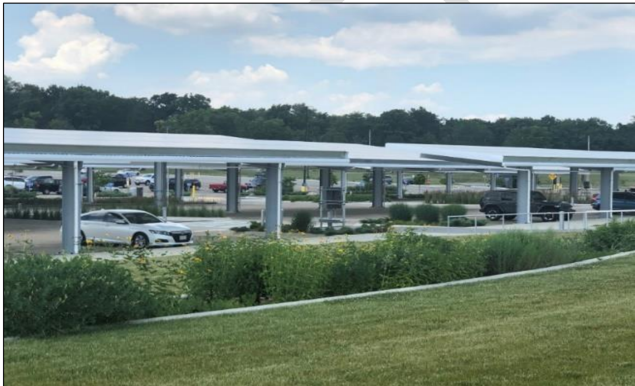
Figure 2-19 – EVV Solar-Covered Lot
