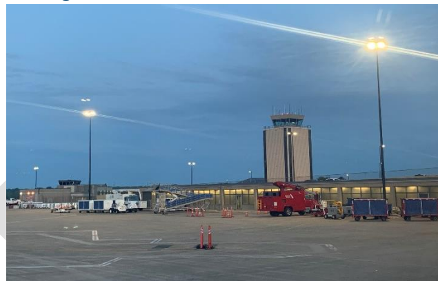
Figure 2-21 – Air Traffic Control Tower
