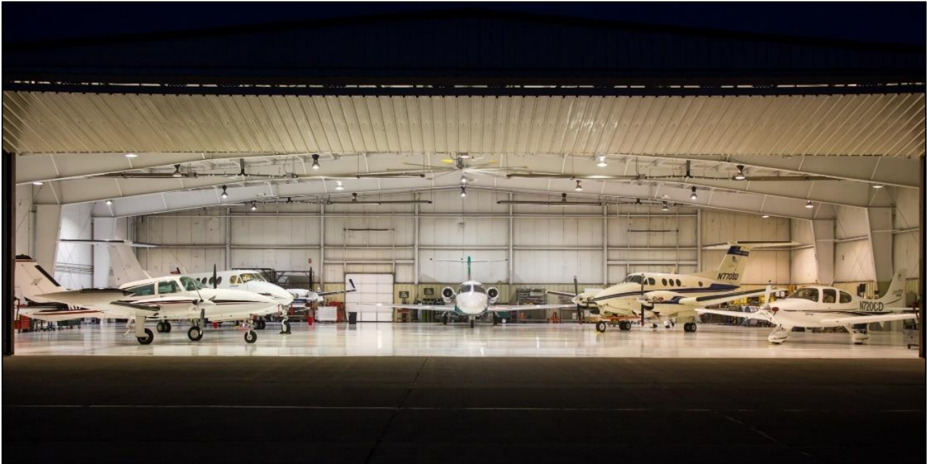
Figure 2-26 – Tri-State Aero Maintenance Hangar
