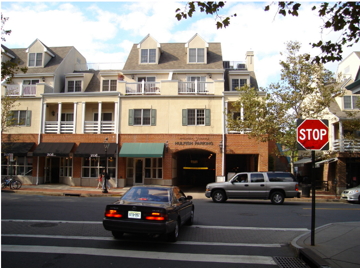
These street-oriented mixed-use buildings obscure the parking structure behind.
