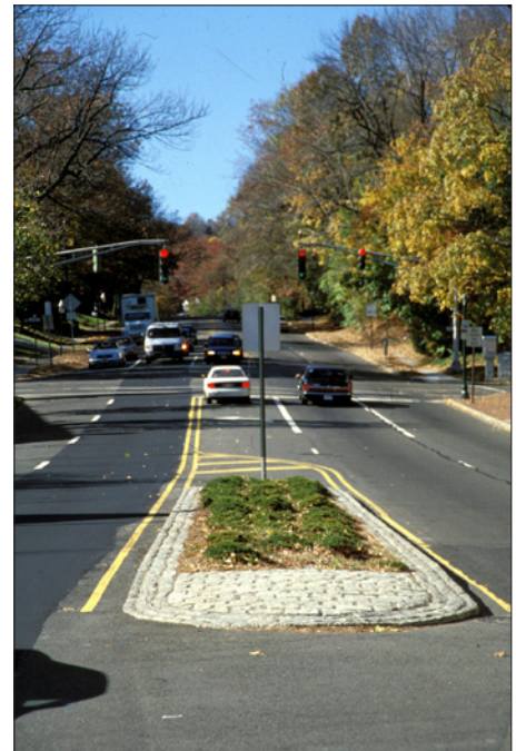
Traffic Calming—landscaped medians and pedestrian refuges.
