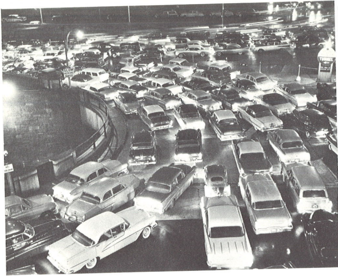
Jam-up entering the Queens-Midtown Tunnel. Between 8 and 9 a.m., 8,000 persons use this facility to enter the central business district while 140,000 enter on the Queens subways and 33,000 on the Long Island Rail Road. A third tube and its Queens approaches would cost $275 million and yet allow less than 3,000 additional persons—2 percent of the peak hour arrivals from Queens—to enter Manhattan between 8 and 9 a.m.
