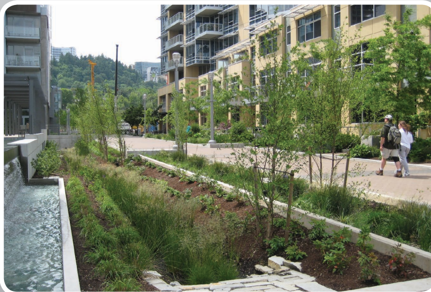
Vegetated shales absorb and filter rain water and stormwater runoff naturally.
