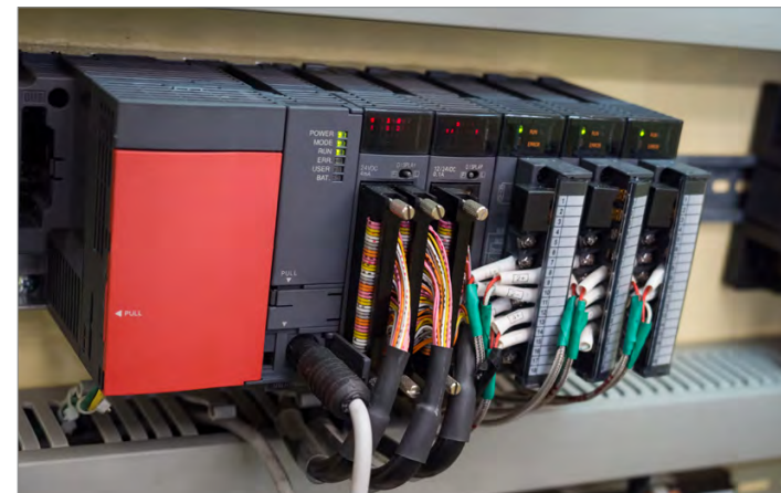
Shown here is a typical PLC installation on DIN rail. Image: Dreamstime
