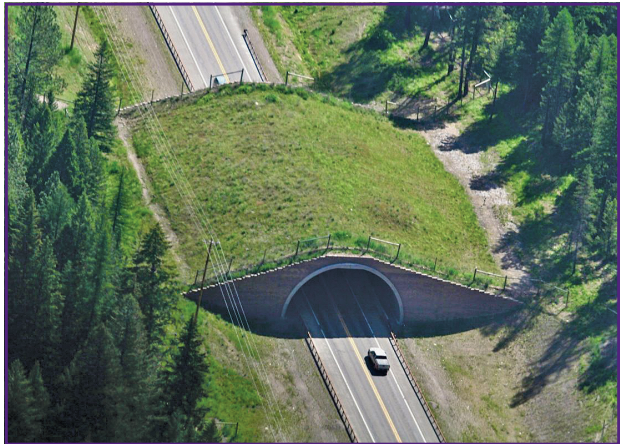
A wildlife overpass along U.S. Highway 93 in Montana. Across 76 miles, US-93 features 81 fish and wildlife crossing structures. Photo Credit: Kylie Paul / CLLC
