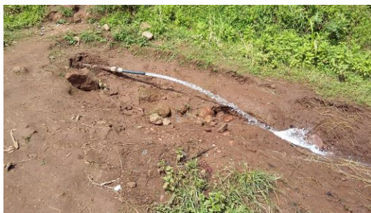
Picture 1 Fractured water supply pipe (HDPE) in Dheshkele Kebele, Bonke Woreda, GG Zone
