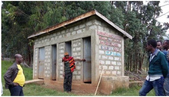
Picture 3 Well constructed school latrine for girls with working doors, incorporating disability access and handwashing facilities, Deshkele Primary School, Bonke Woreda, GG Zone
