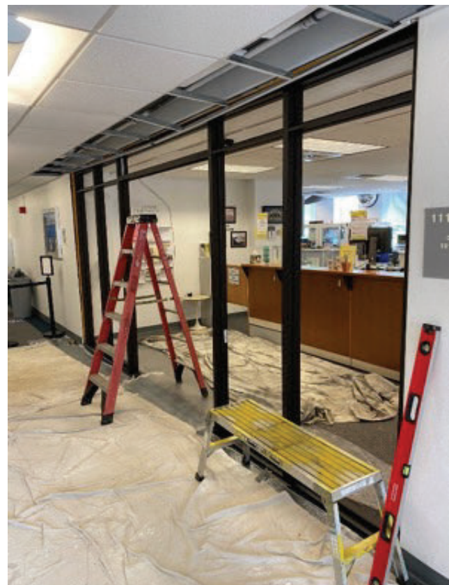
New electrified storefront doors being installed by a Justice Systems' subcontractor to retrofit an access control system. Justice Systems performs as prime contractor on the majority of our projects – giving the agency a single-point of responsibility for coordination and overall performance.
