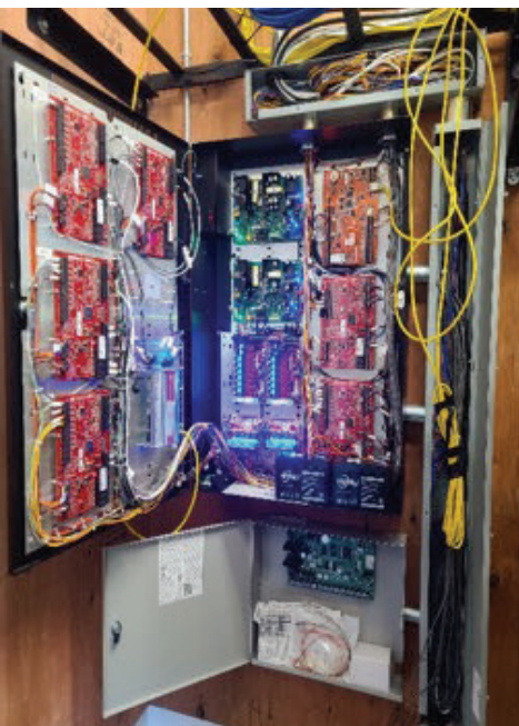
Burglar alarm/ intrusion / panic alarm panel beneath the access control panel at Island County Camano
