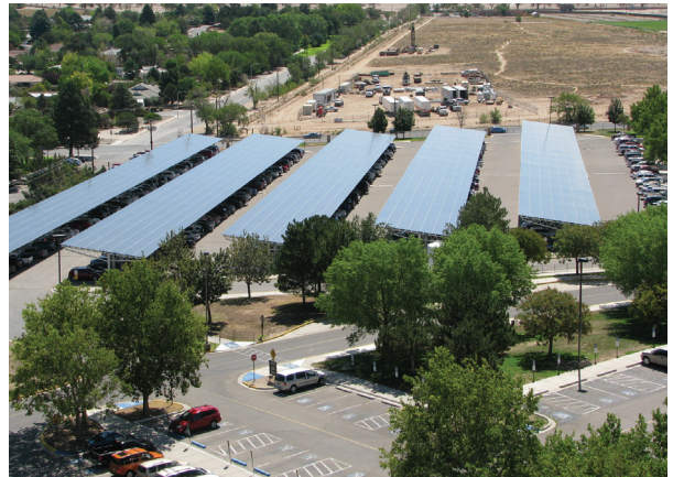
A parking lot for doctors and nurses at the VA healthcare facility in Albuquerque now includes solar panels to provide a design capacity of 1,016 kW.
