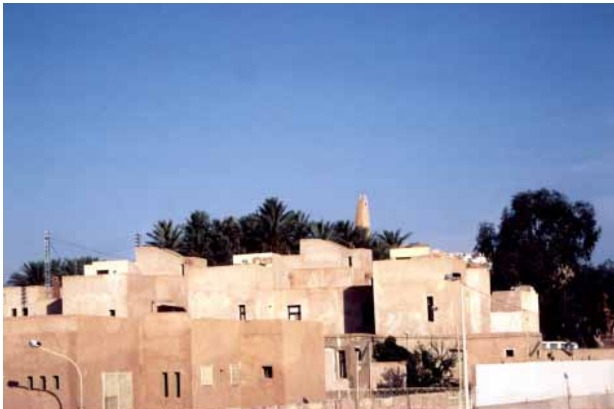
Detail. Facades are rendered with traditional mortar
