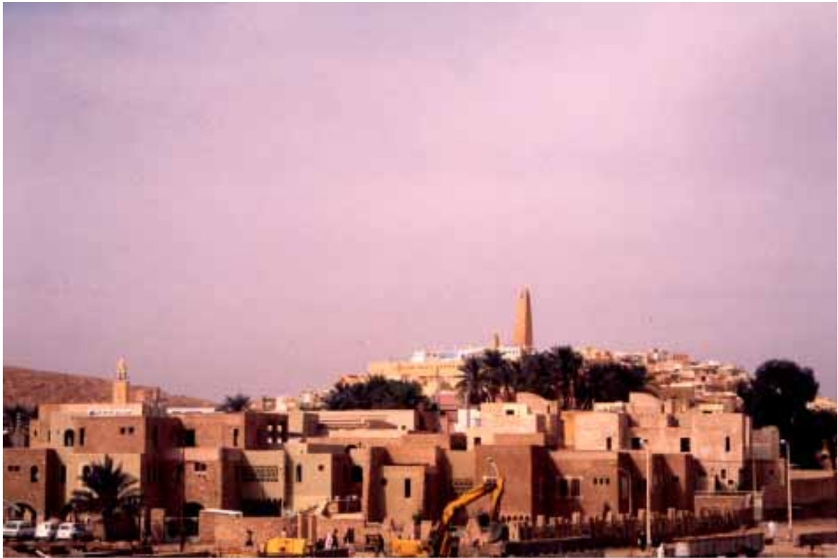
General view, with the town of Ghardaia in the background
