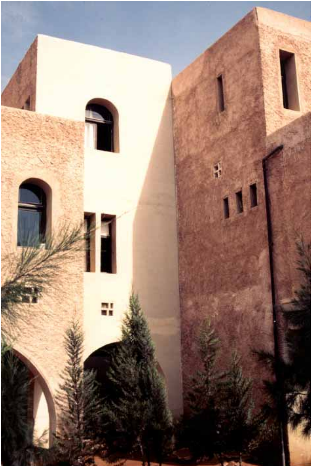
Openings on faade are minimal, in reaction to climatic constraints
