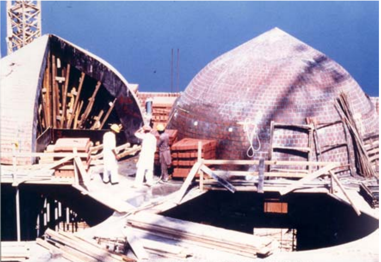
Juffali Mosque: Prayer Hall Domes during Construction
