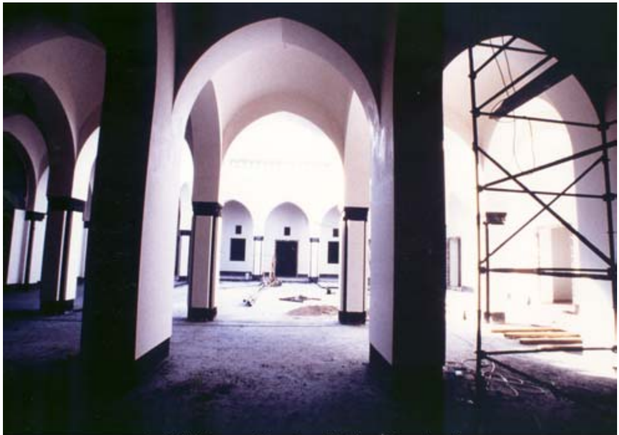
Juffali Mosque: Courtyard during Construction
