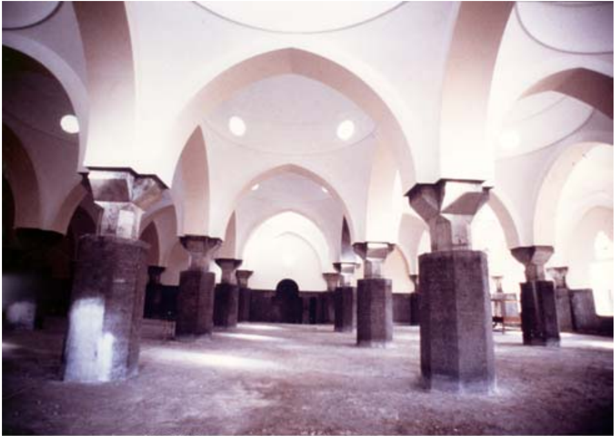
Juffali Mosque: Prayer Hall during Construction
