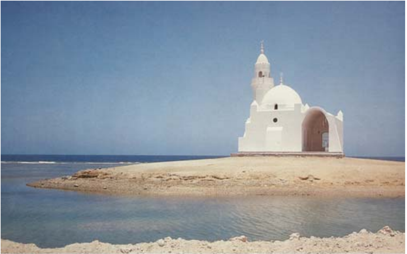
Corniche Mosque: Overall View
