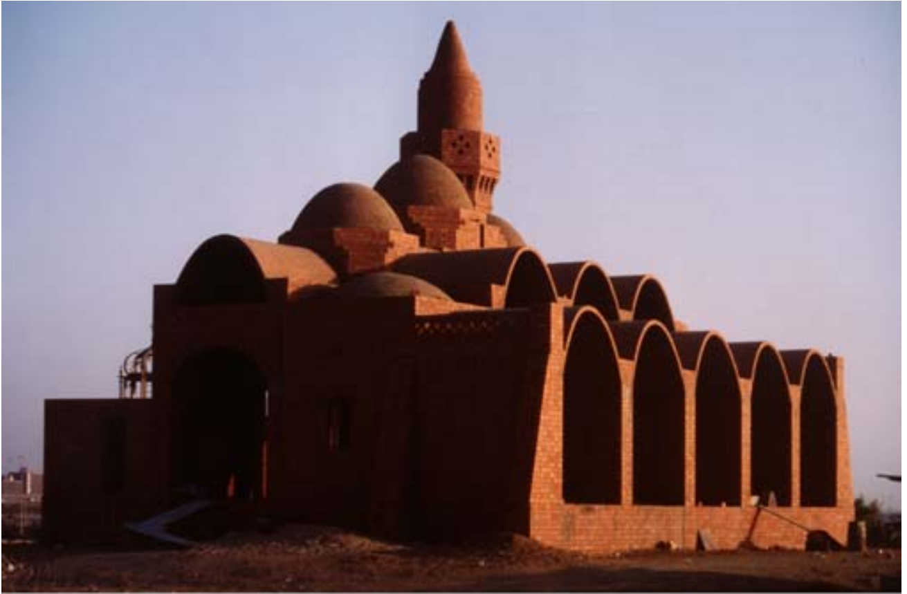
Ruwais Mosque during Construction
