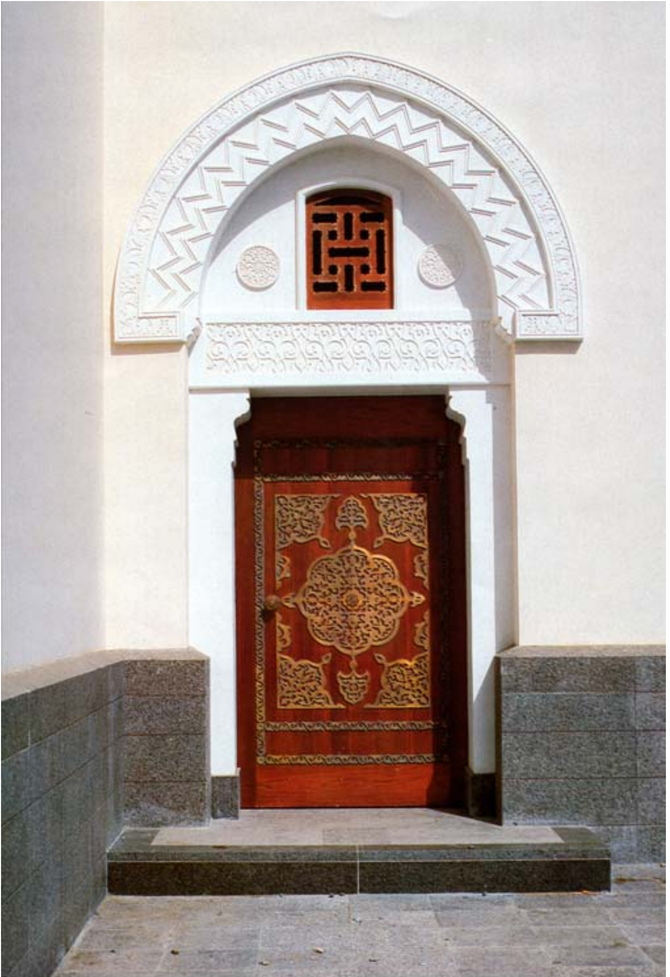
Island Mosque: Door in Teakwood and Brass
