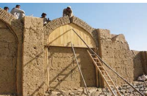
Reconstructing mud-brick arches between pakhsa piers in the perimeter wall.
