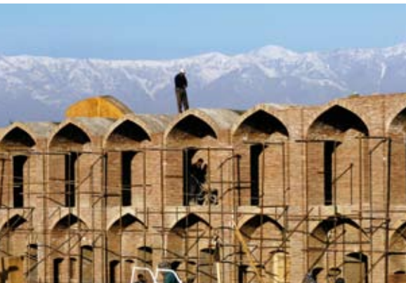
The new caravanserai complex uses traditional brick-masonry techniques. Below, the building near completion.
