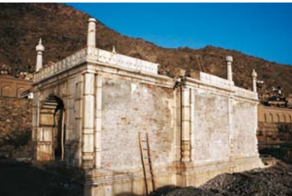
The west elevation of the Shahjahan Mosque prior to and during replacement (below) of the marble facing.
