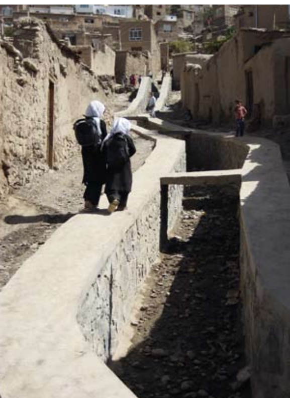
Newly built storm-water drain with pathways in the informal settlement on the slope above Baghe Babur.
