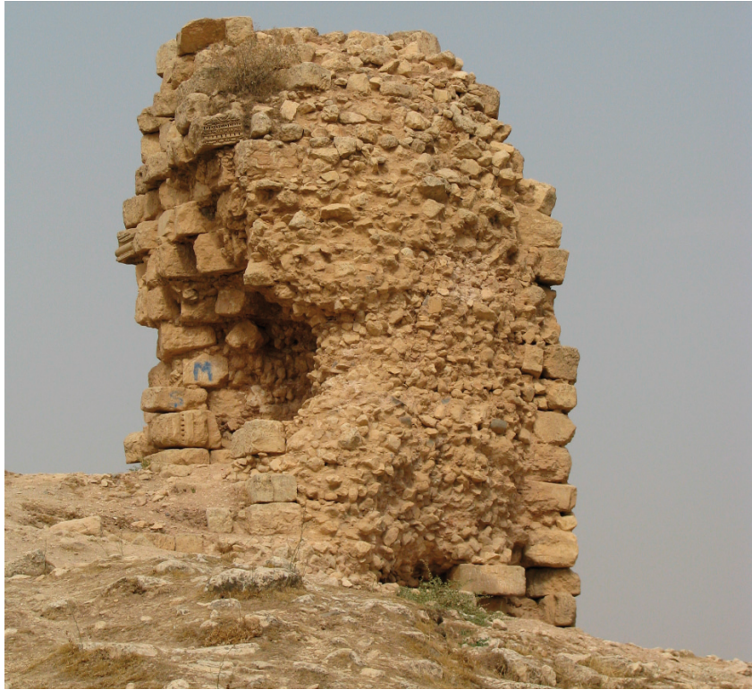
Fig. 5. Urfa, Byzantine material reused in the masonry of a tower of the citadel. (Photo: Mattia Guidetti)
