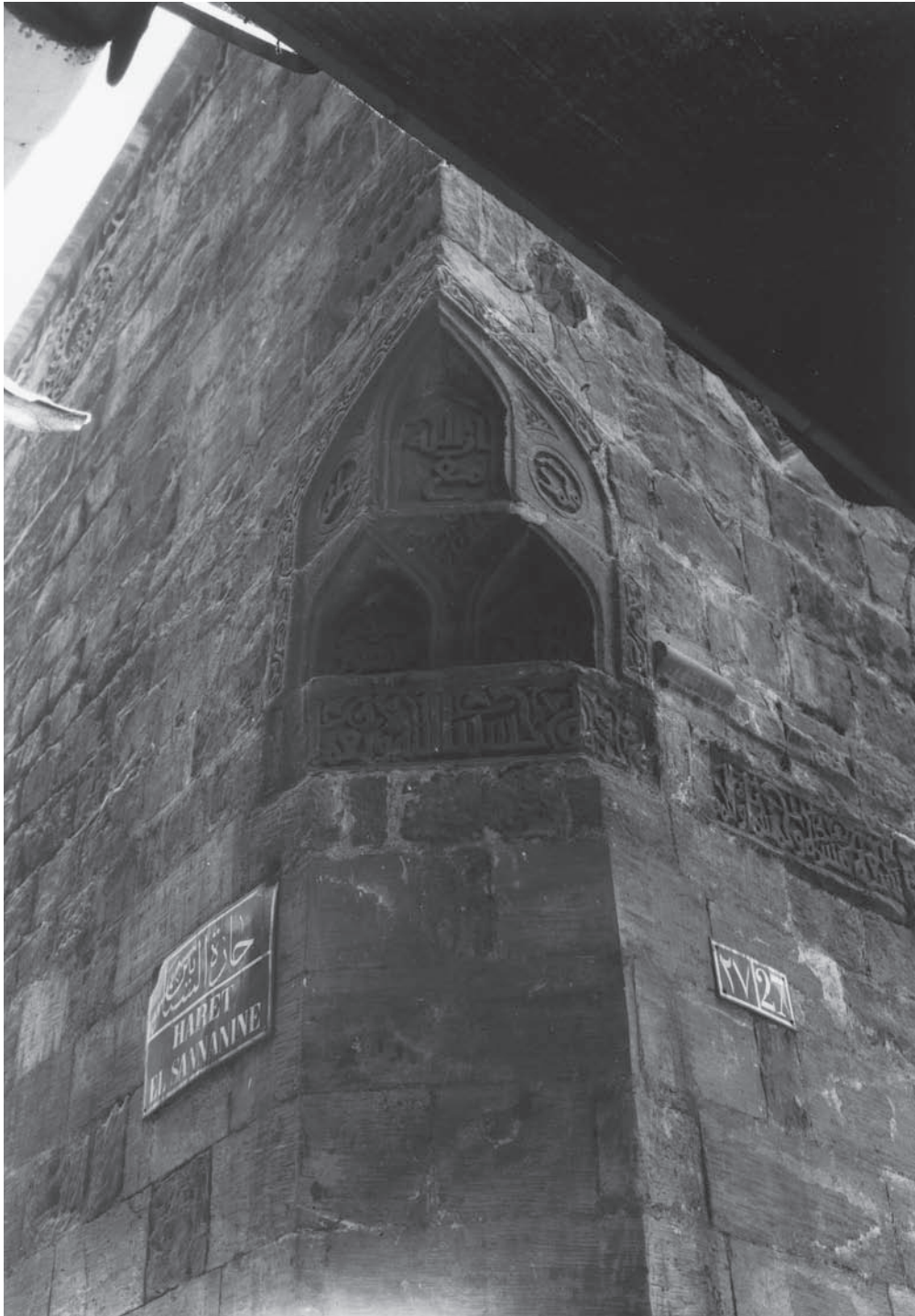
Fig. 9. Mosque of al-Aqmar, 1125, facade. Chamfered corner crowned with keel-arched muqarnas. (Photo: K. A. C. Creswell, © Creswell Archive, Ashmolean Museum, Oxford, neg. no. C. 3890)
