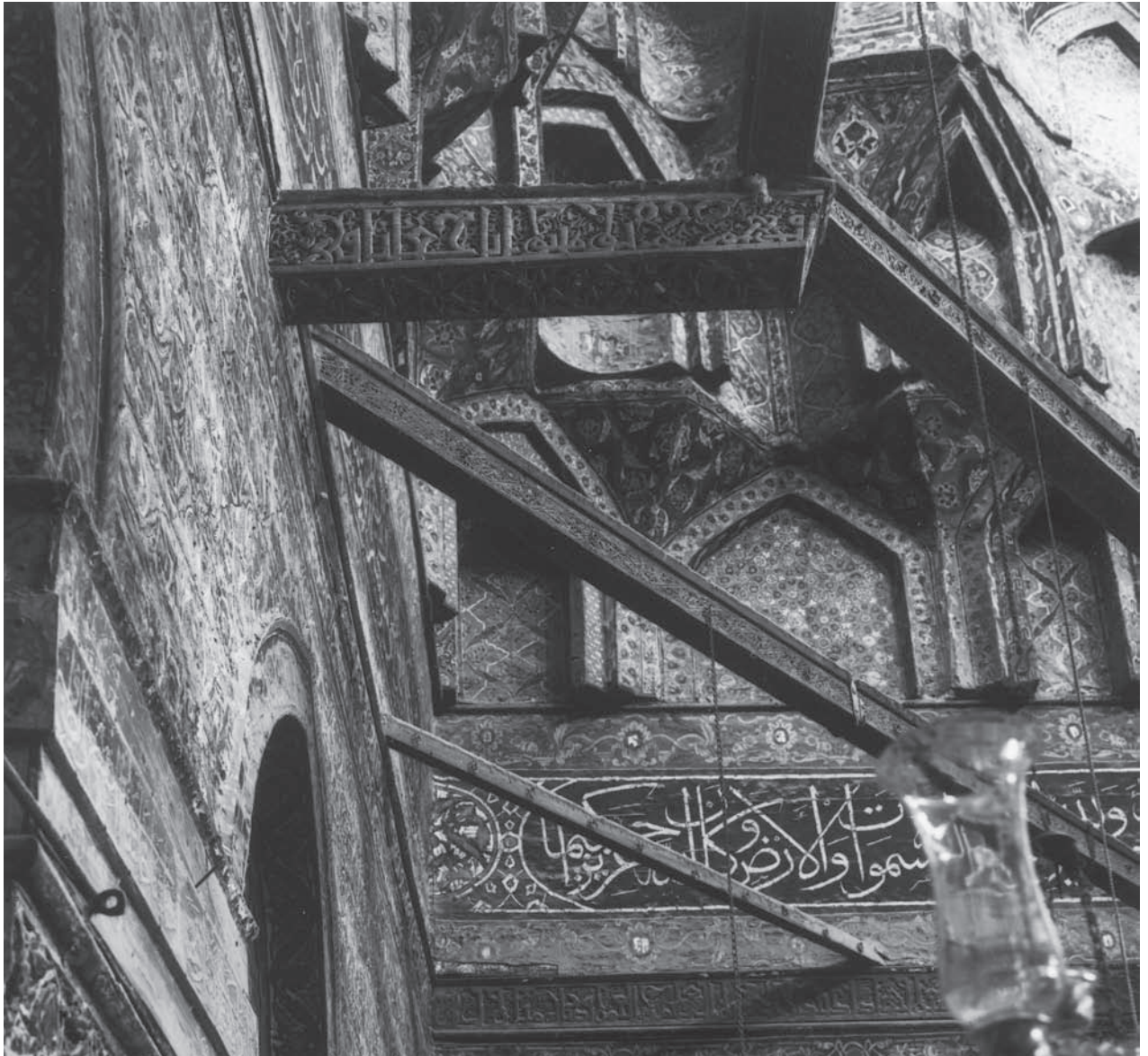
Fig. 6. Mausoleum of Imam al-Shafi'i, interior. Original carved wooden brackets supporting wooden octagon for suspension of lamps. (Photo: K. A. C. Creswell, © Creswell Archive, Ashmolean Museum, Oxford, neg. no. C. 1037)
