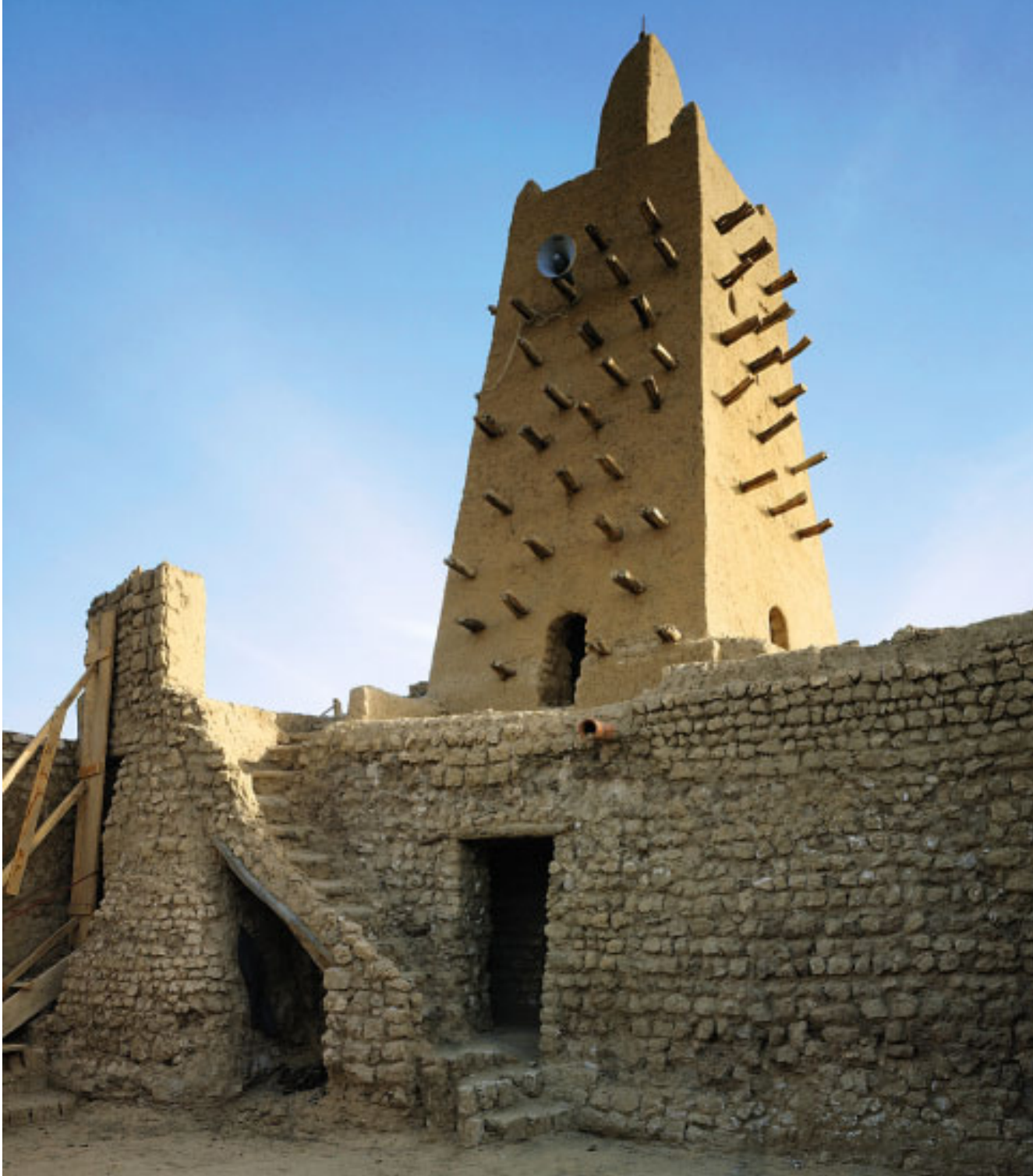
A minaret of Djingareyber Mosque after restoration. The Mosque was built in mud and tuff stone, evident in the foreground of the shot.
