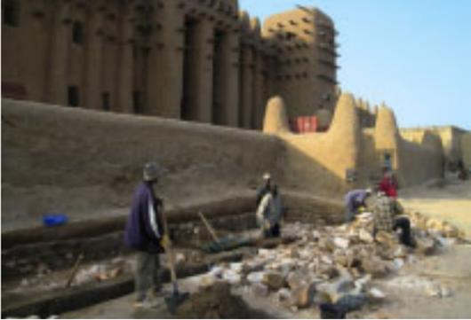
Outside the walls of the Great Mosque of Djenné, Mali, workers construct a pit for the preparation of *banco* – a manually mixed construction material made of clay soil, sand and various straw and organic additives – on the construction site.
