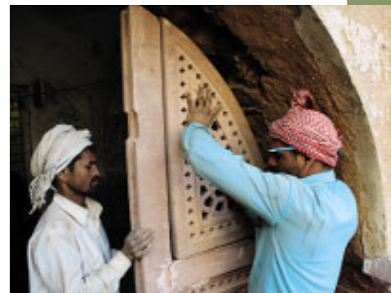
Craftsmen are fitting sandstone jali screens at the Baoli.
