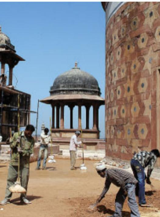
During 2008 and early 2009 over a million kilos of concrete were removed from the roof terrace of Humayun's Tomb.
