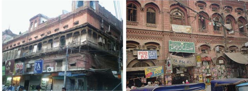
Figure 15 and 16: Adaptive reforms. An old building at Anarkali enameled by the web of electric wires and billboards. (Source: Authors).
