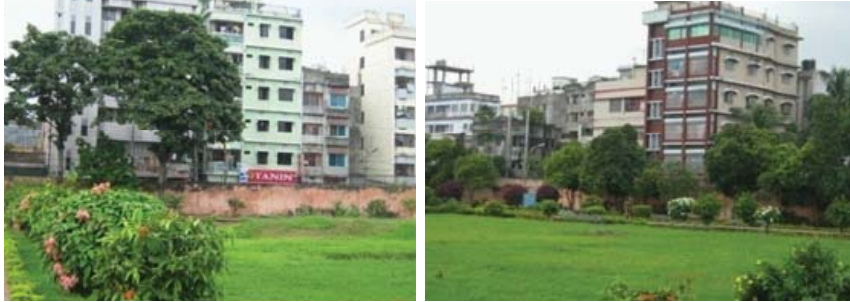
Figures 7 and 8: Incompatible height of the adjacent buildings causes visual obstruction to the fort complex (Source: Authors).
