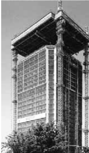
Figure 3: Big Canopy – Automated Construction System for High-Rise Buildings (Thai Obayashi, www.thaiobayashi.co.th ).
