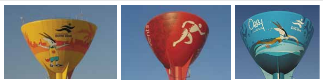
Figure 1-g: Decorated water towers in different colors acted as landmarks that define different urban districts within the city of Doha. (Source: A. Hasanin).
