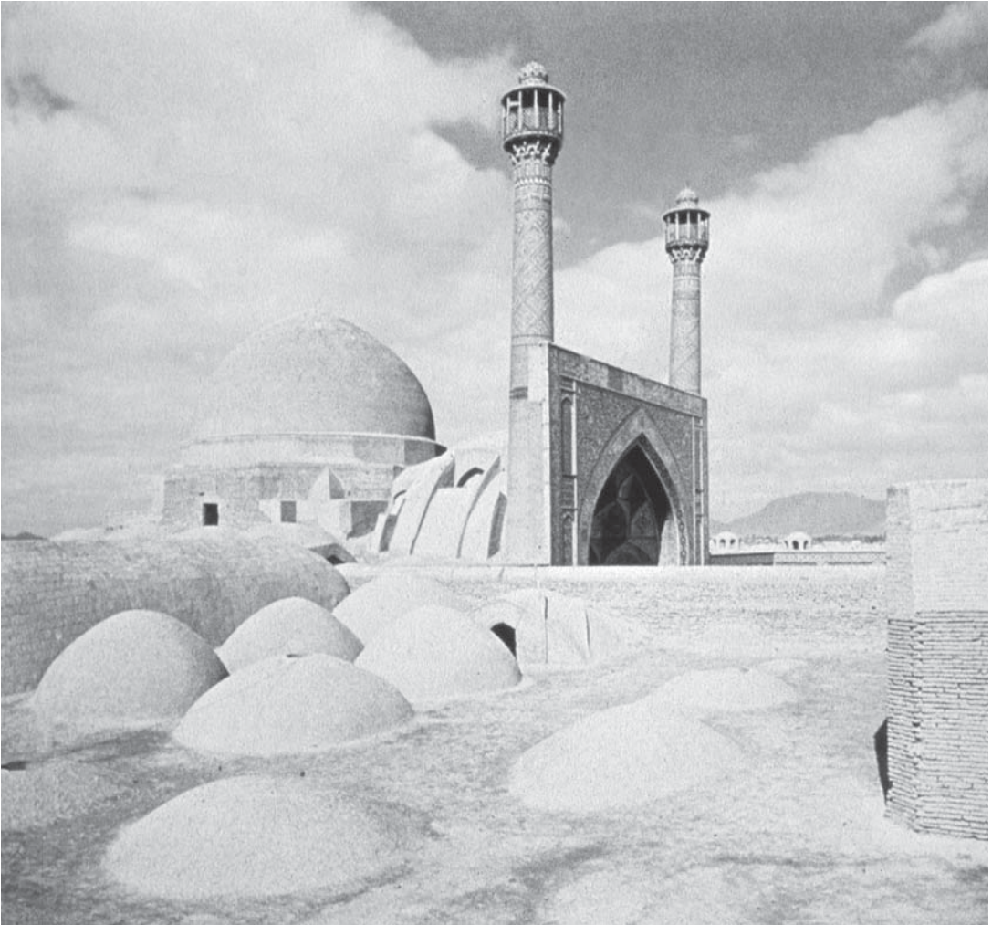
6 Southern dome of Seljuq mosque, Isfahan
