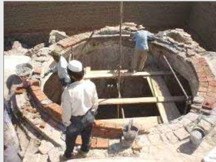
Re-building of a brick masonry dome using traditional techniques
