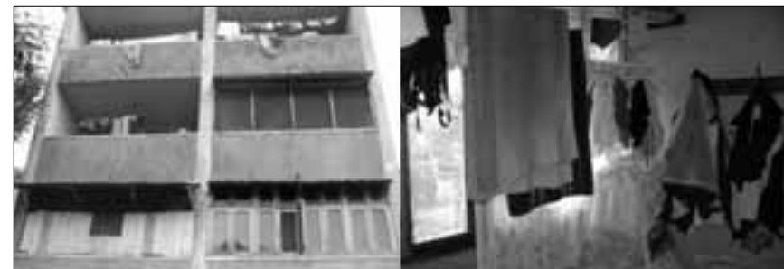
fig 9 A balcony is wholly enclosed by a wall to form a habitable space. (source: Author, 2005)
