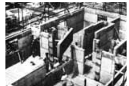
fig 2 Prefabricated panel construction of Praunheim Siedlung (source: ref. 15)
