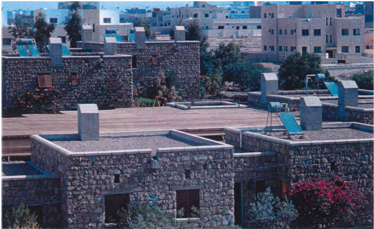
Above: The buildings were constructed using natural stone available in the mountains surrounding the city of Aqaba. The stone was not mechanically cut or dressed but left completely rough.
