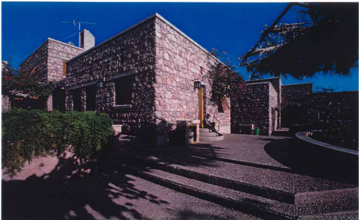
Above: The buildings were constructed using natural stone available in the mountains surrounding the city of Aqaba. The stone was not mechanically cut or dressed but left completely rough.
