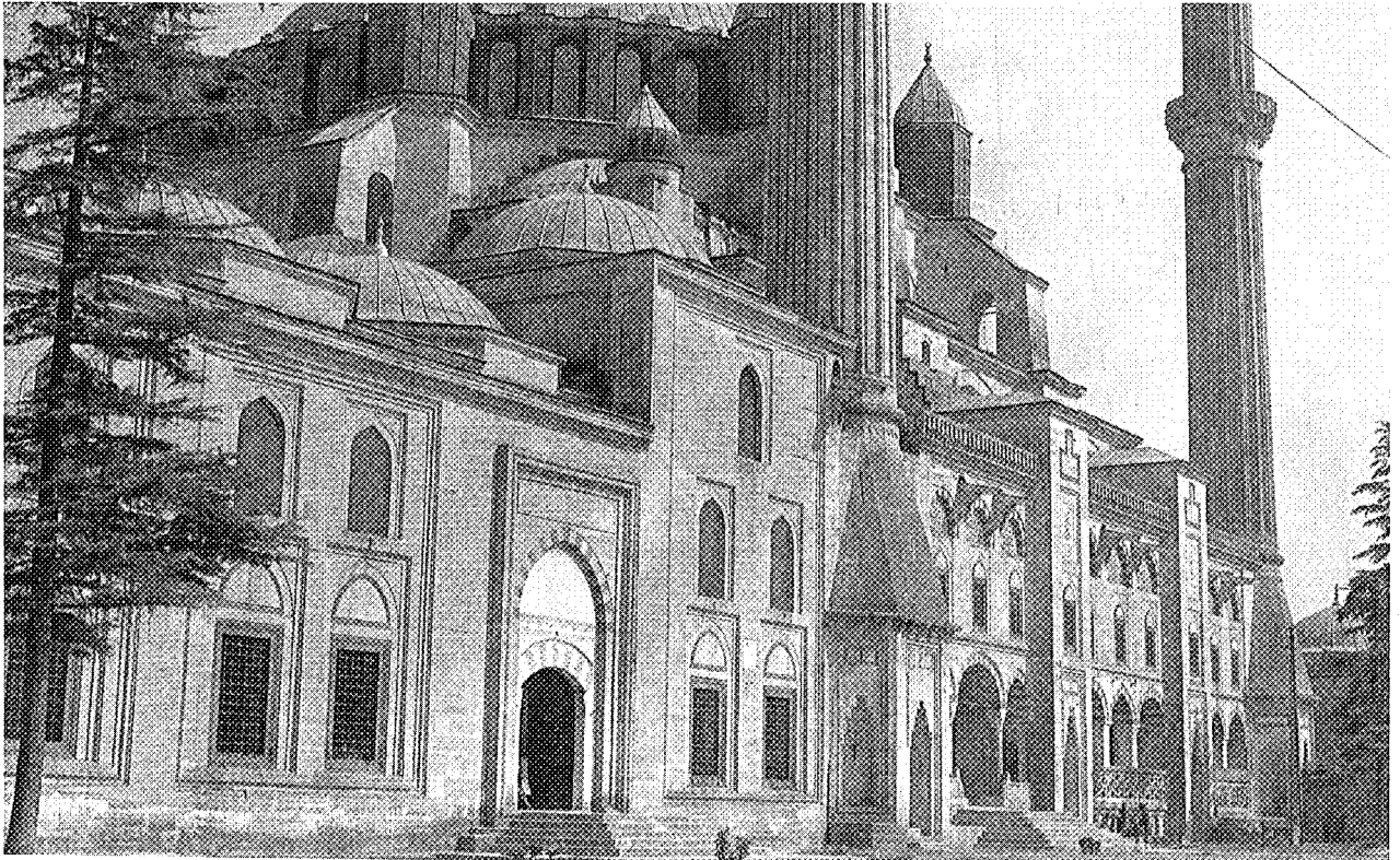
17. Side view of the Selimiye mosque.
