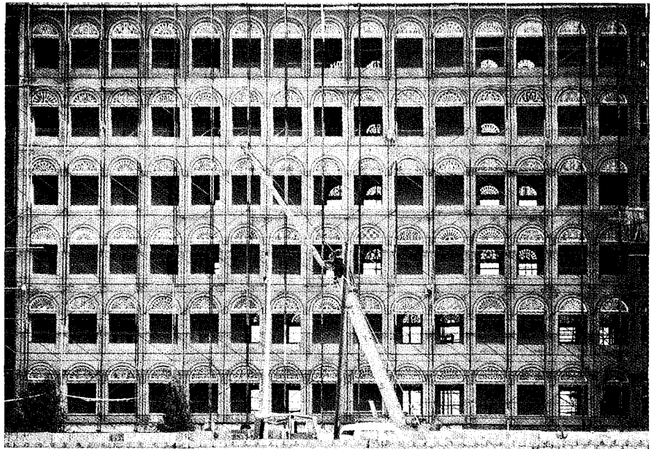
A new construction in Sana'a using precast floor height panels.
