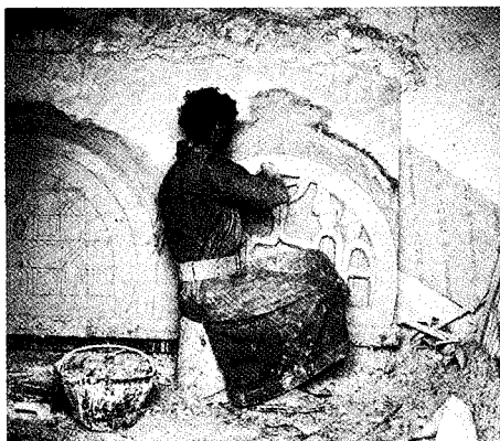
A craftsman making a gypsum window according to traditional methods.
