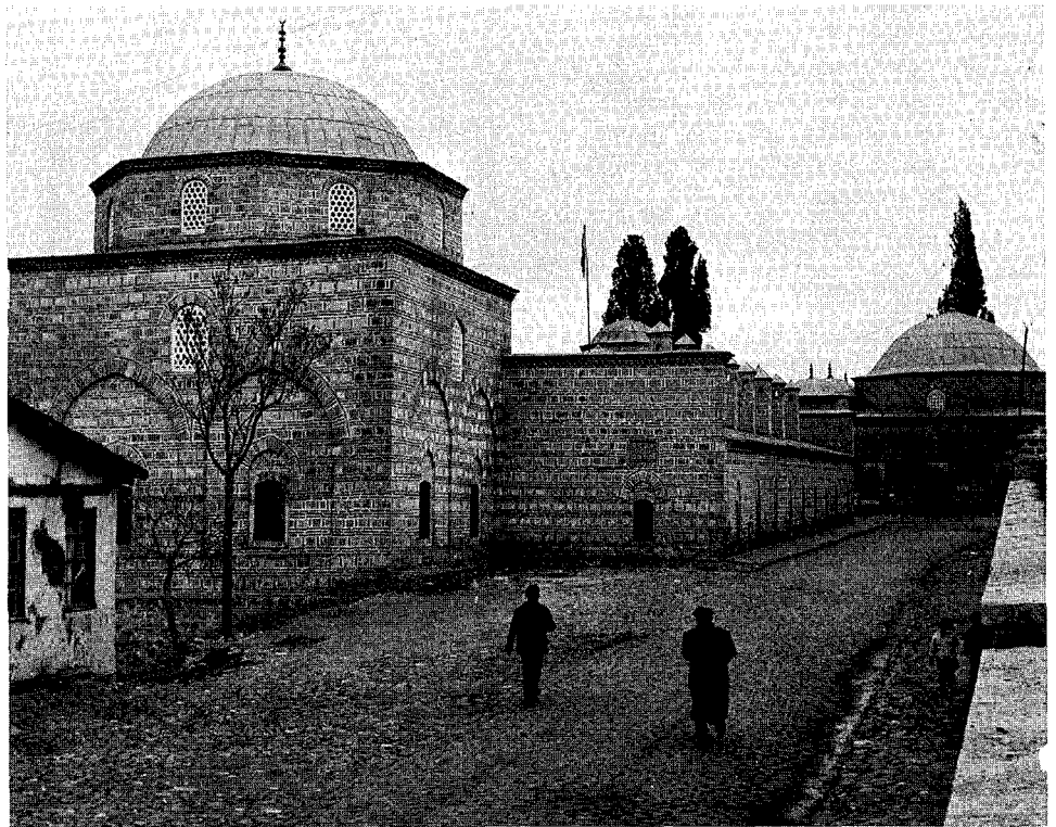
Bursa, Madrasa of Yıldırım Bayezid, late 14th century—an early Ottoman madrasa, constructed of stone and brick courses. The classroom, in the form of a domed eyvan, protrudes from the building mass both horizontally and vertically
