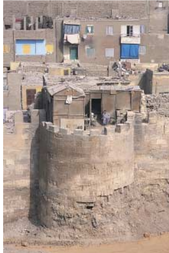
Illegal encroachments on the Ayyubid wall.
