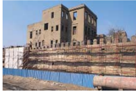
Above: Darb Shoughlan school facility under rehabilitation.
