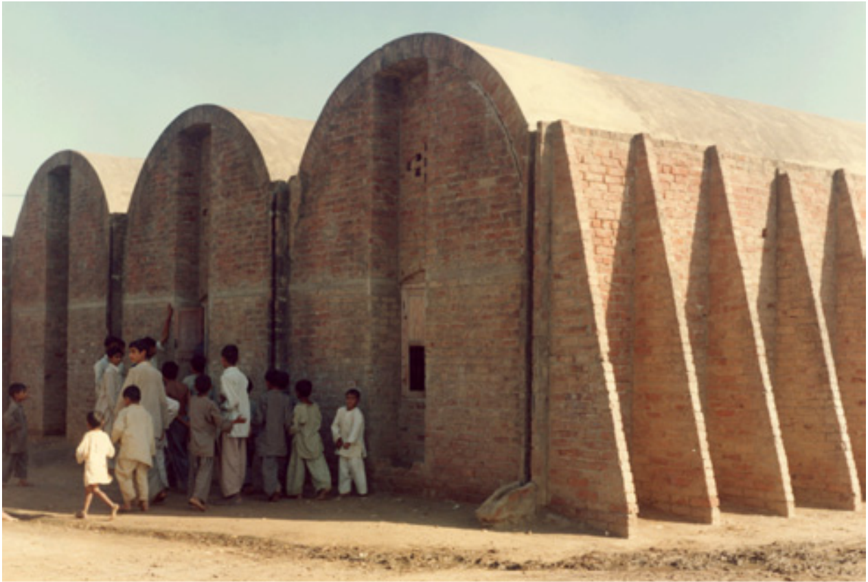
Storage shed modified to serve as three-room school. Village council financed half the cost.
