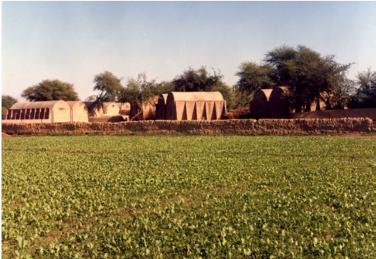
The farmer's house. Behind parapet the flat roof above vaults for use as roof terrace.
