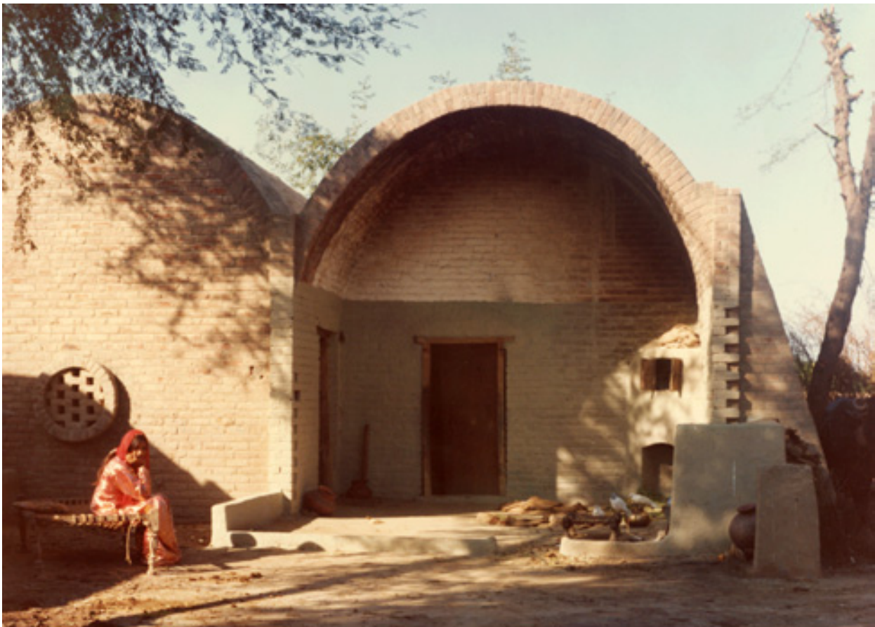
Openings shaded from sun by overhang, or kept small and screened with brick djallis
