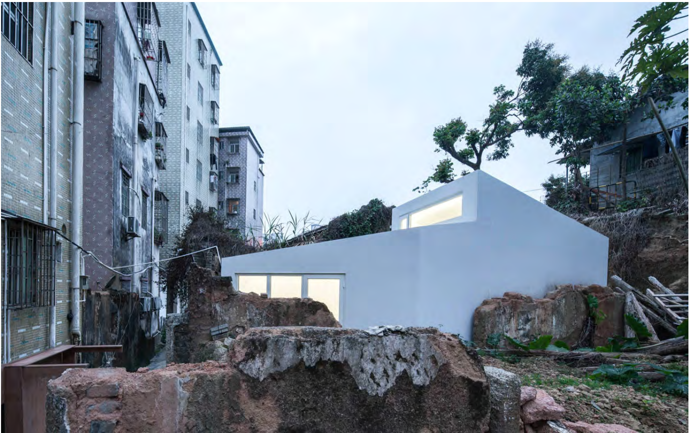
Plugin in Shenzhen. The Plugin system allows to upgrade, renovate and replace damaged old structures without demolishing historic buildings and relocating families. It is a way of preserving historic traces in old structures.
