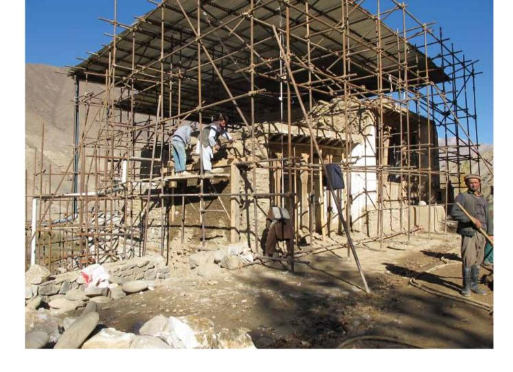
Conservation work entailed the removal of debris and re-roofing of the shrine, a delicate measure considering the highly decorated woodwork used to construct its ceiling.
