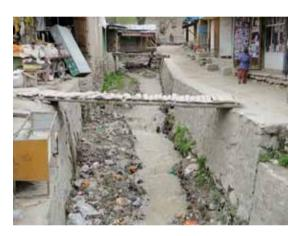
Storm-water drains in the old town are poorly maintained and often become blocked due to dumping of commercial waste.
