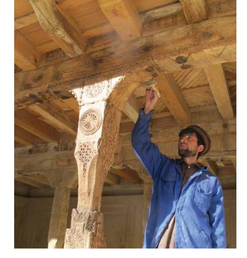
Right, linseed oil was applied to areas of woodwork to prevent damage from moisture.
