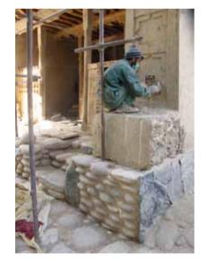
Above, external elevations were cleaned and repaired, before being finished with a mixture of mud-gypsum plaster.
