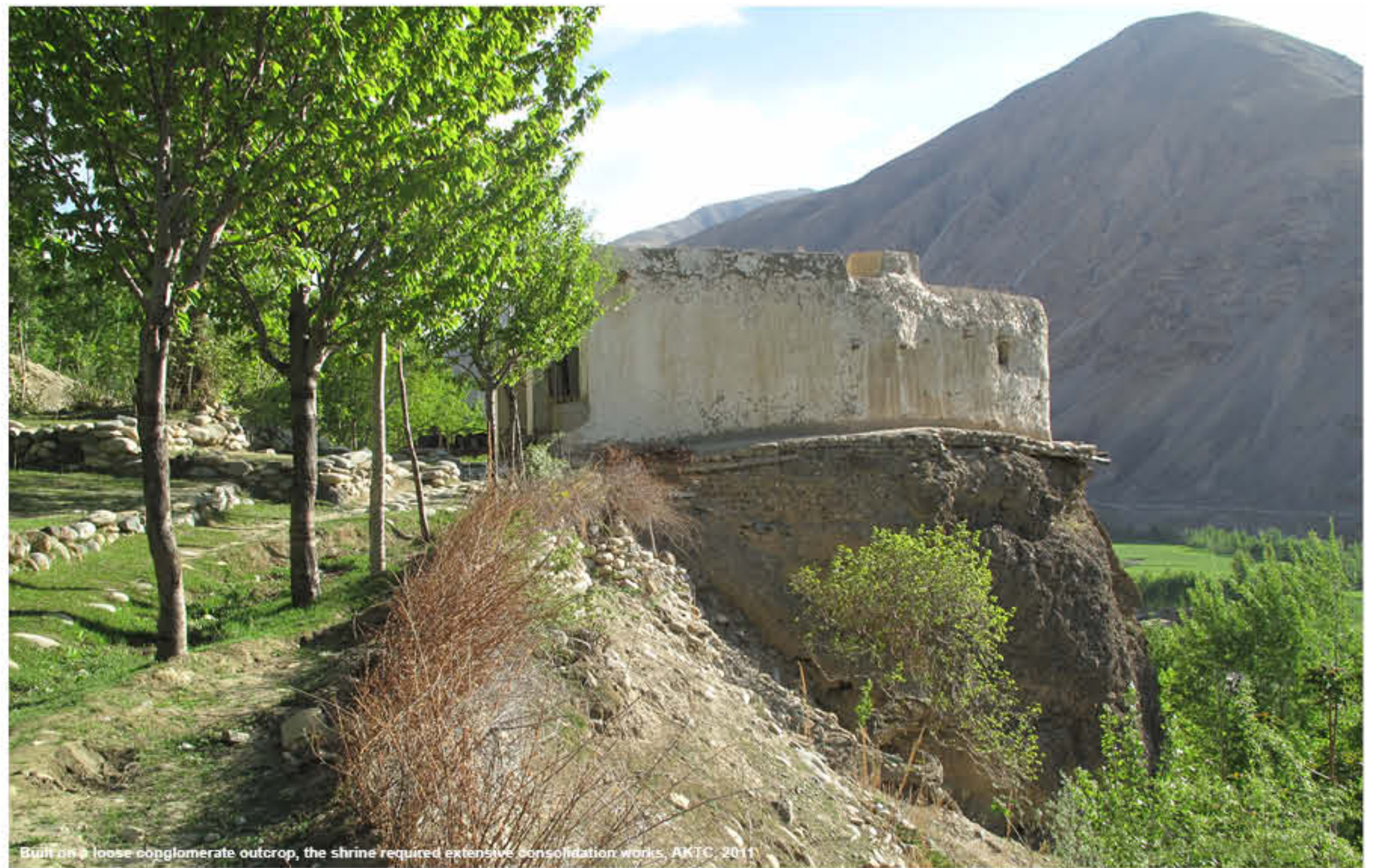
Building's loose conglomerate outcrop, the shrine required extensive consolidation works, AKTC, 2011
