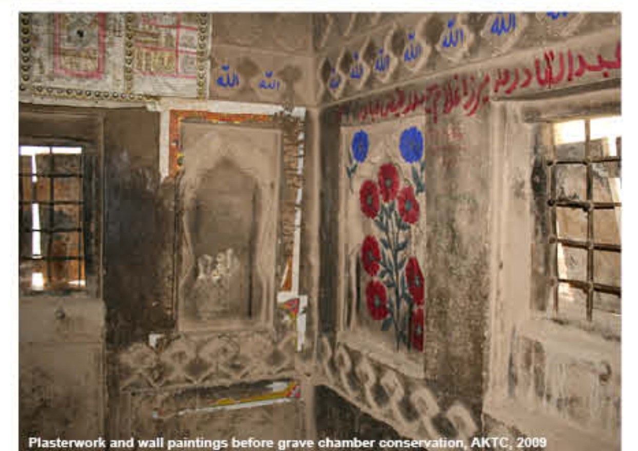
Plasterwork and wall paintings before grave chamber conservation, AKTC, 2009
