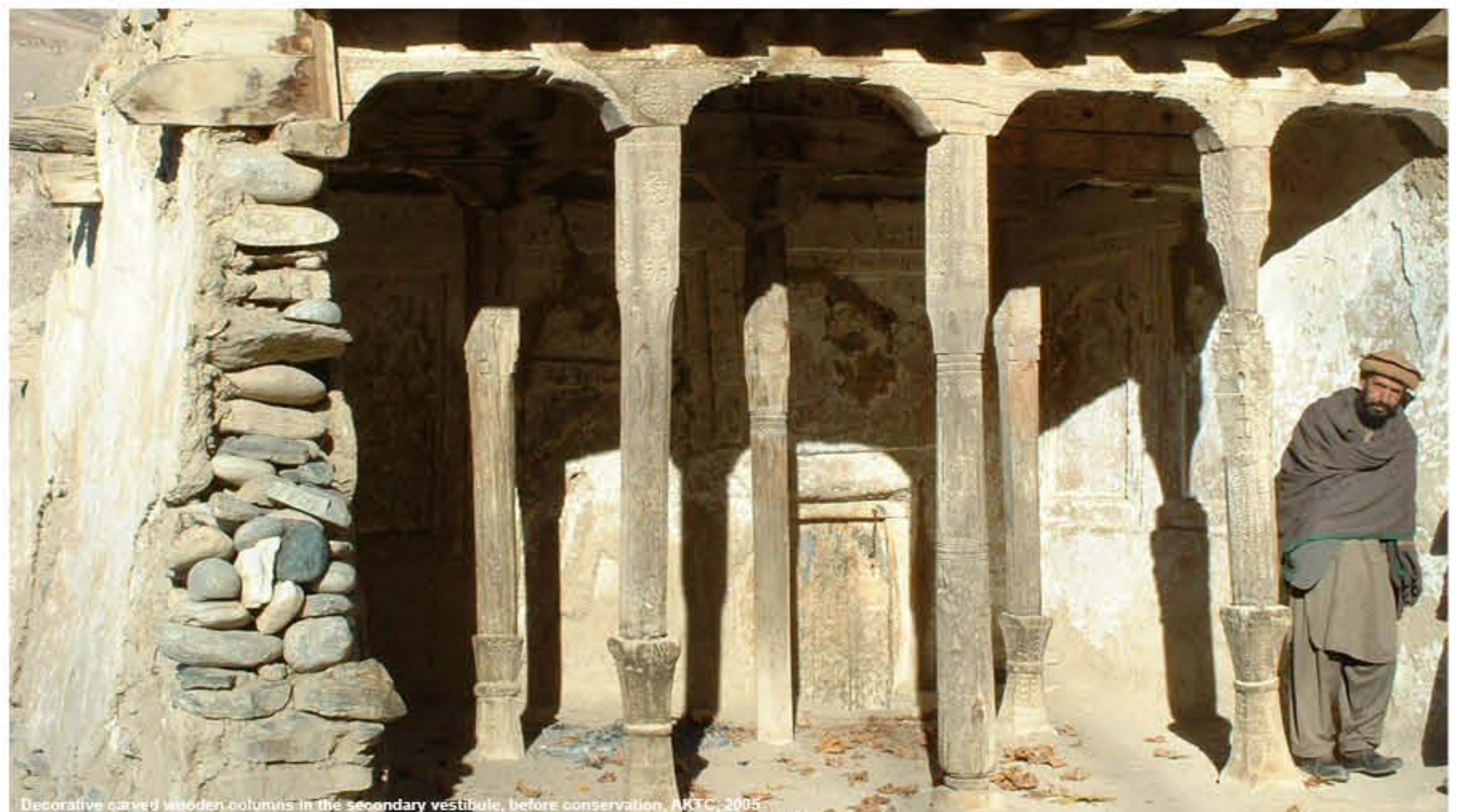
Decorative carved wooden columns in the secondary vestibule, before conservation, AKTC, 2005
