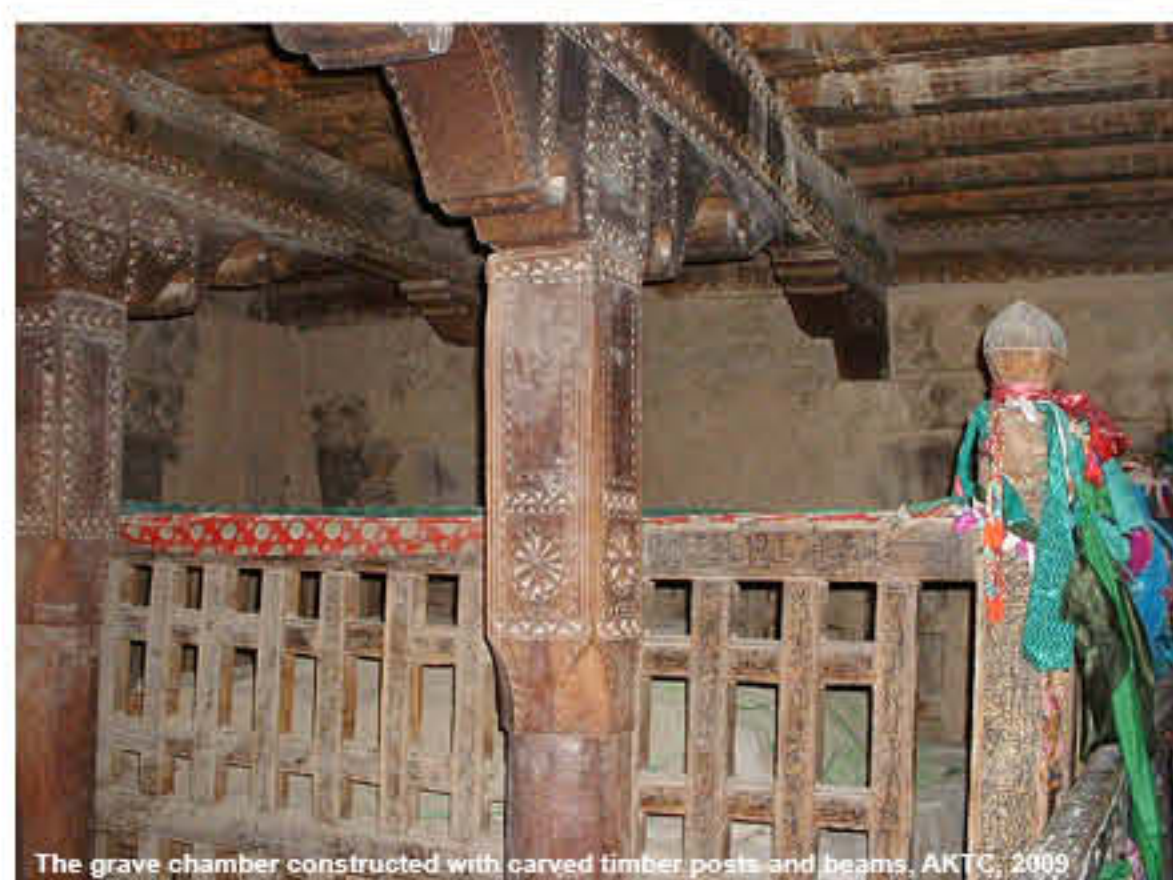
The grave chamber constructed with carved timber posts and beams, AKTC, 2009
