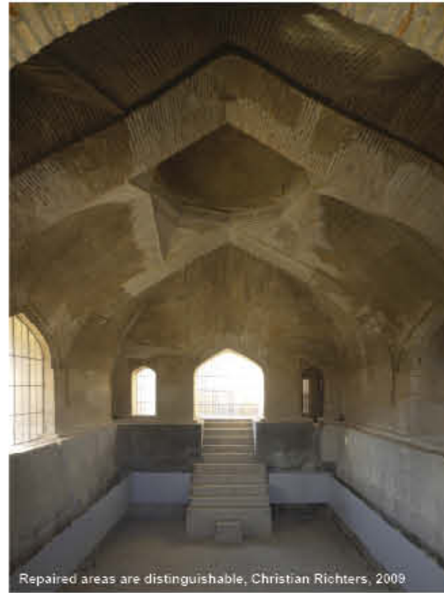
Repaired areas are distinguishable, Christian Richters, 2009
