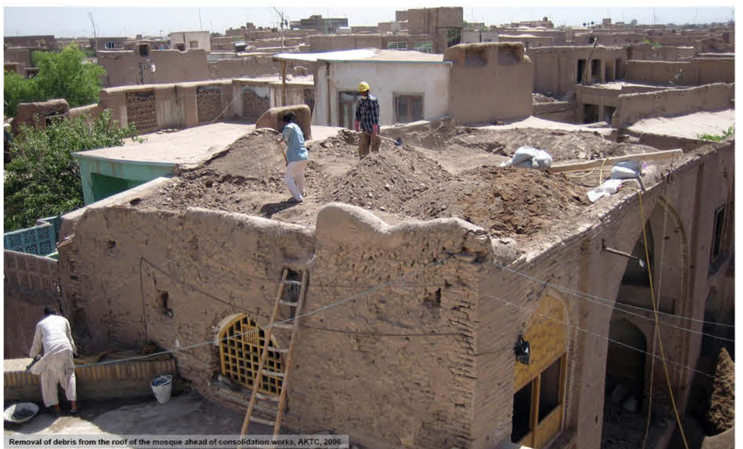
Removal of debris from the roof of the mosque ahead of consolidation works, AKTC, 2006
