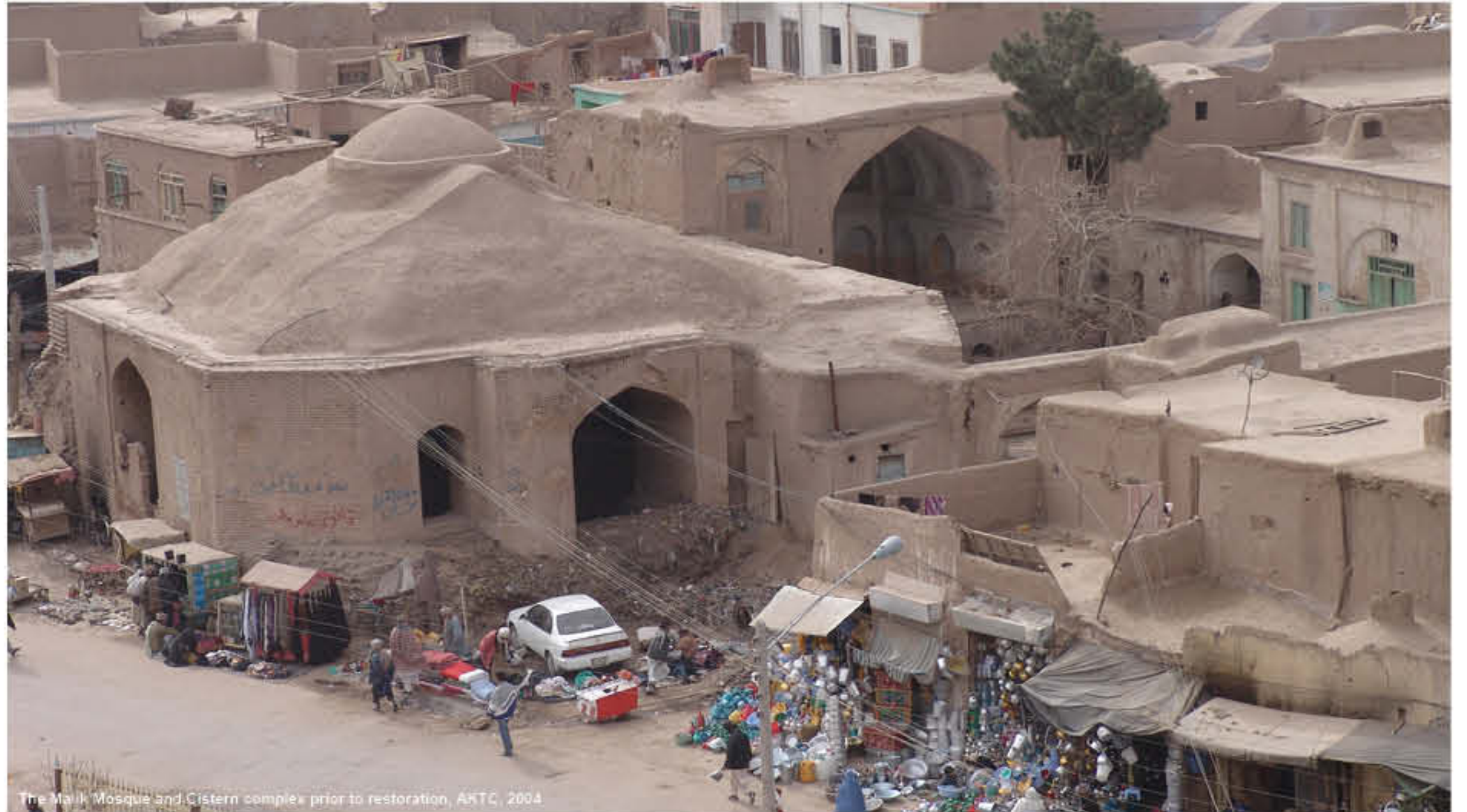
The Malik Mosque and Cistern complex prior to restoration, AKTC, 2004
