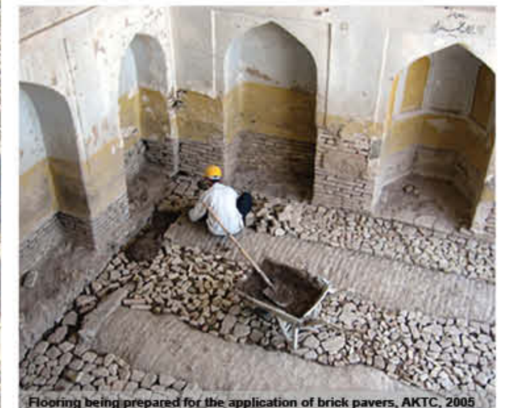
Flooring being prepared for the application of brick pavers, AKTC, 2005
