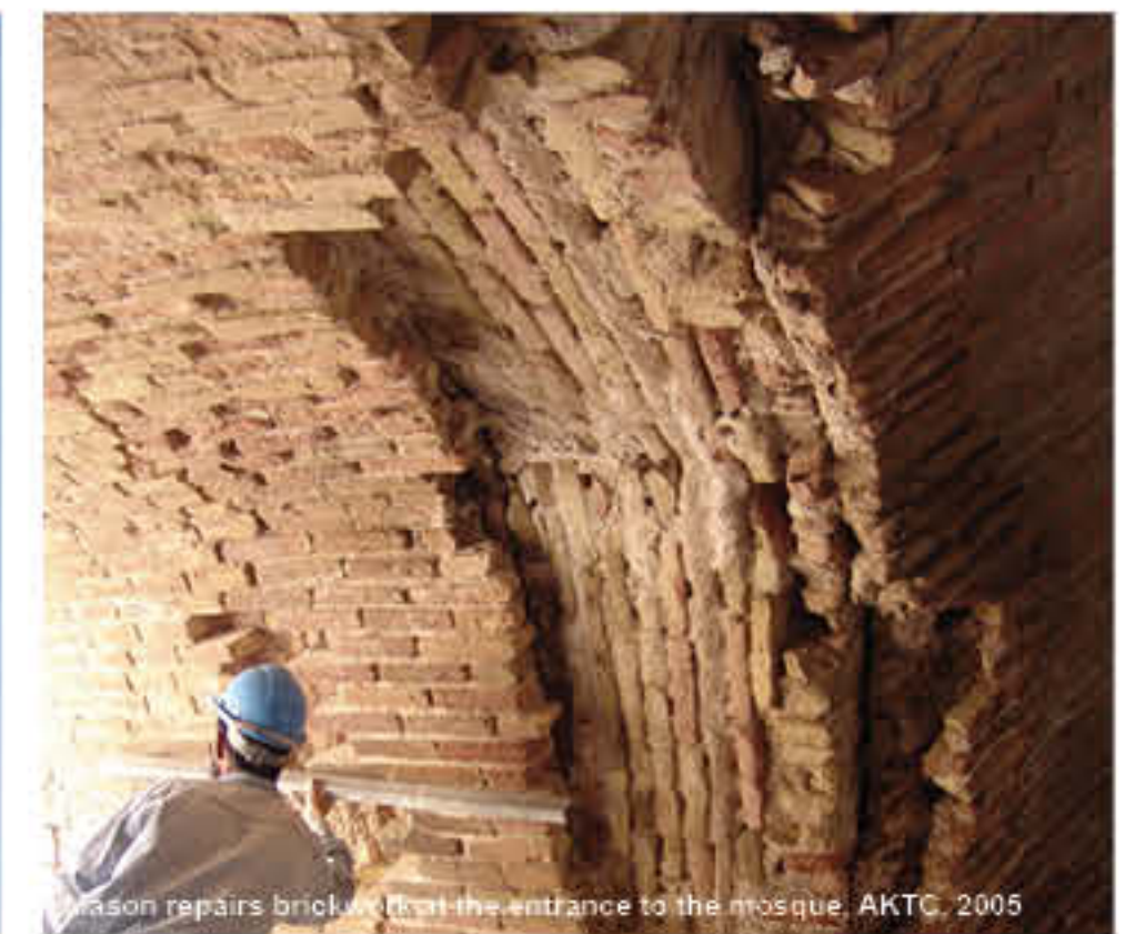
Mason repairs bricks at the entrance to the mosque, AKTC, 2005
