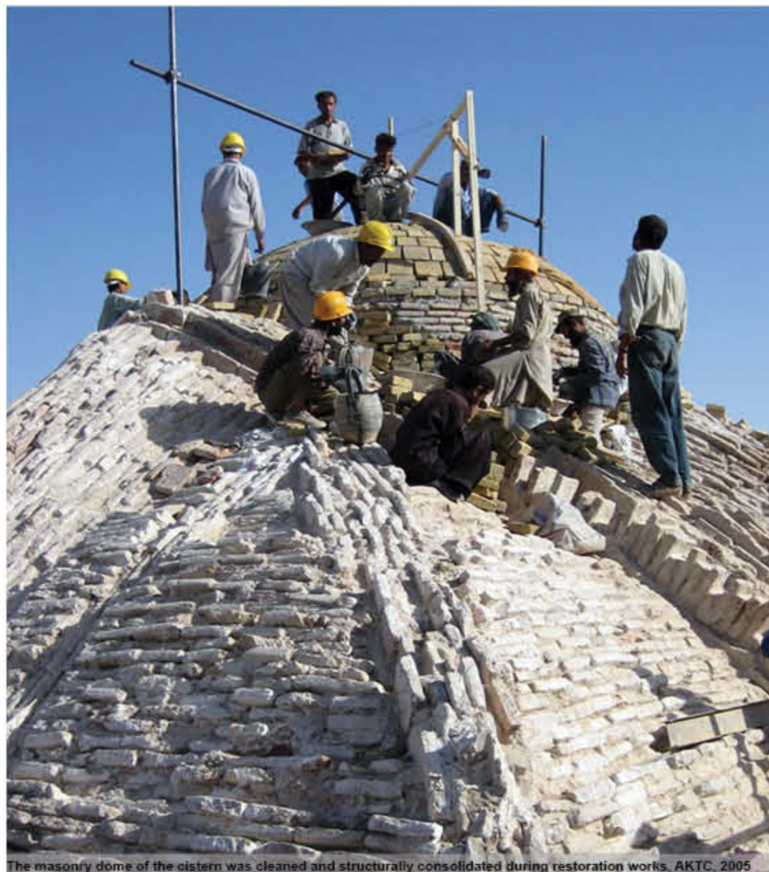
The masonry dome of the cistern was cleaned and structurally consolidated during restoration works, AKTC, 2005
