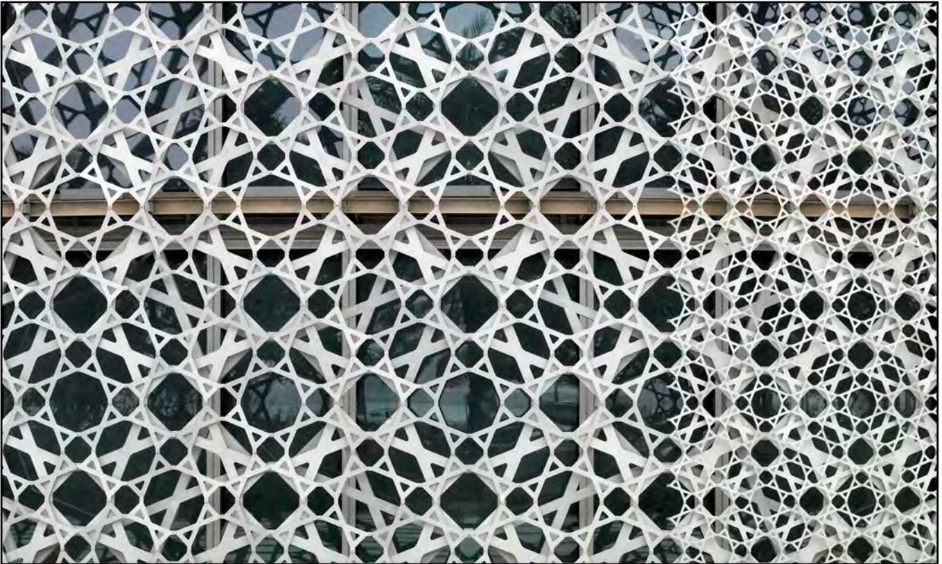
The facade's screen pattern is comprised of aluminium "butterflies" at four different scales. This brise-soleil screen, inspired by the traditional Islamic mashrabiyya. The geometric pattern at several scales is overlaid at different densities along the facade in response to the solar conditions.
