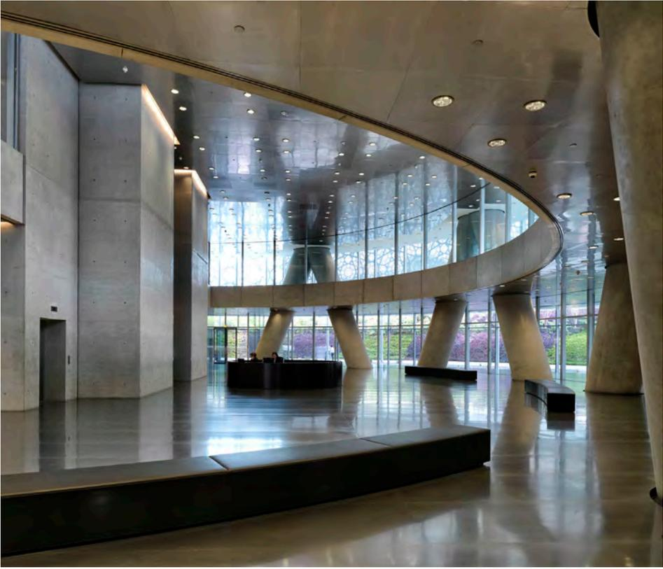
The primary vertical load of the building is placed on a diagrid “tube” of canted round columns forming an X-shaped structural frame at the perimeter of the circular floor plan.
