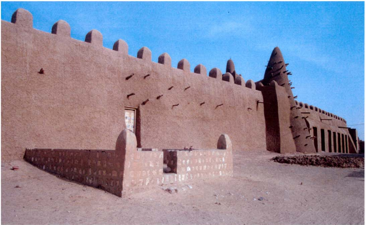
Above: South door and parapet built in "alhore" or limestone.
