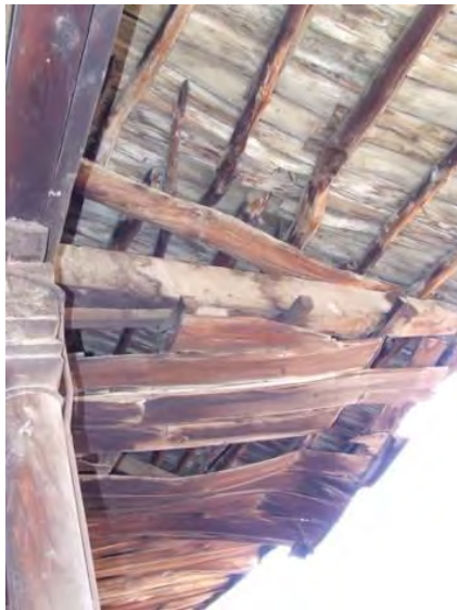
Figure 22. Case04 Deterioration Problems of the Roof (left) and Floor (right) (Color change) (Source: Authors, 2008).
