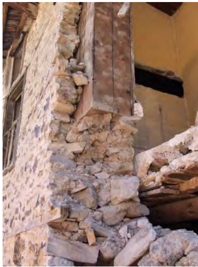
Figure 6. (Left) and Figure 7. (Right) Masonry and Wooden Frame (Hımış) Wall Examples (Source: Authors, 2008).
